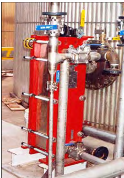
Adhesive Manufacturer Formaldehyde Cooler MODU-FLEX™ Model MFK022 - 2" ports Design Pressure: 150 PSIG Heat Transfer Area: ~ 200 ft 2
