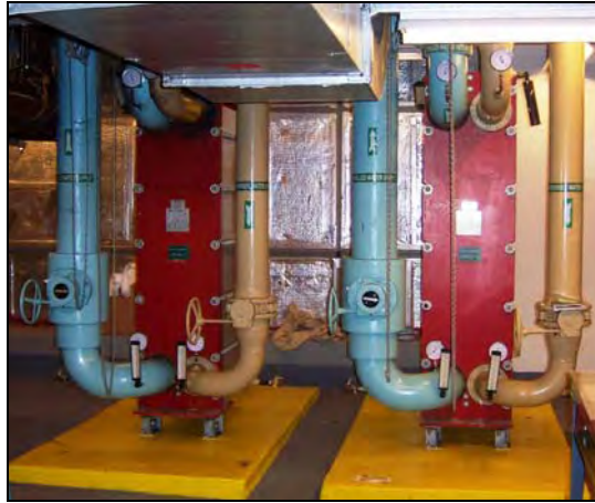
NYC Mid-Town Hotel Free Cooling Exchangers MODU-FLEX™ Model MFK063 - 6" ports Three in Parallel Design Pressure: 300 PSIG Heat Transfer Area: ~ 2,200 ft 2
