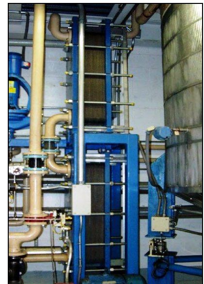
Specialty Oil Processor Batch Cooler & Heater MODU-FLEX™ Model MFK043 - 4" ports Design Pressure: 150 PSIG Heat Transfer Area: ~ 350 ft 2
