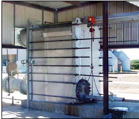
Southern Power Plant Closed Water Exchanger MODU-FLEX™ Model MFK201 - 20" ports Design Pressure: 150 PSIG Heat Transfer Area: ~ 8,000 ft 2
