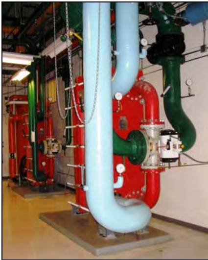
Major US City Business Center Condenser Water Cooler MODU-FLEX™ Model MFK081 - 8" ports With Diverter Valve & Control Design Pressure: 300 PSIG Heat Transfer Area: ~ 3,000 ft 2
