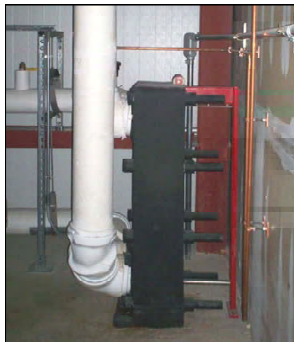
Chocolate Processor Process Water Cooler MODU-FLEX™ Model MFK042 - 4" ports Design Pressure: 150 PSIG Heat Transfer Area: ~ 125 ft 2
