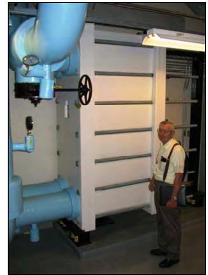
Modern Hotel Chilled Water Exchanger MODU-FLEX™ Model MFK082 - 8" ports Design Pressure: 300 PSIG Heat Transfer Area: ~ 5,200 ft 2
