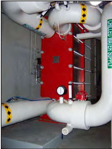
New York Business Center Chiller By-Pass MODU-FLEX™ Model MFK084 - 8" ports One of Three Units Design Pressure: 300 PSIG Heat Transfer Area: 4000+ ft 2
