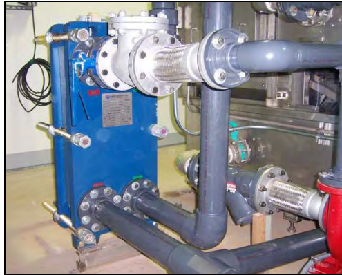
Food Processing Plant Enzyme Temperature Control MODU-FLEX™ Model MFL041 - 4" ports Design Pressure: 150 PSIG Heat Transfer Area: ~ 300 ft 2
