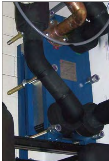
Computer Chip Manufacturer Batch H Cooler MODU-FLEX™ Model MFK021 - 2" ports Design Pressure: 150 PSIG Heat Transfer Area: ~ 25 ft 2
